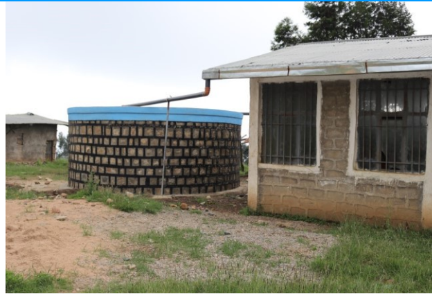
50 m3 roof rain water harvesting reservoir constructed at Kufanzik primary school
