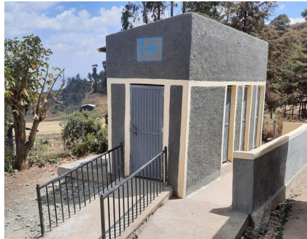
Latrine construction at Kufanzik health center
