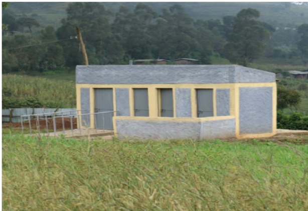
School latrine constructed at Kufanzik Primary
