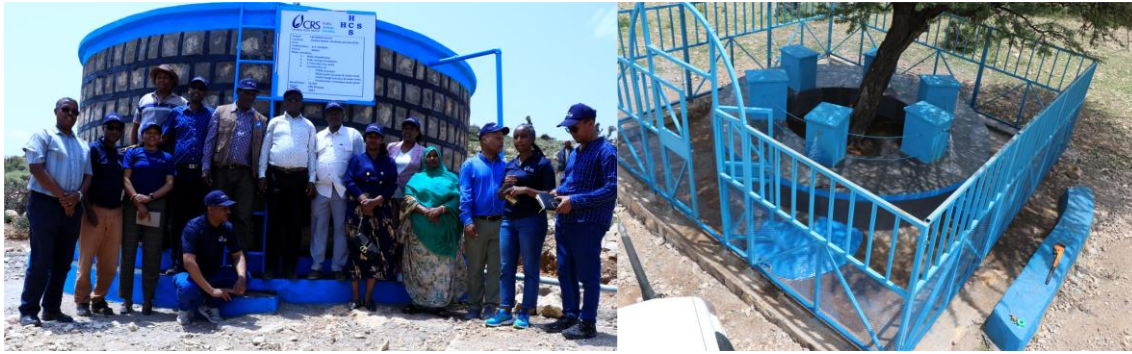
Figure 18: Bodley Reservoir and water point constructed in Somali Region
