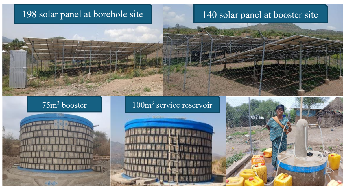
Figure 15: Solar-powered water supply at Wedeti Kebele in Chiro woreda, West Harerghe
